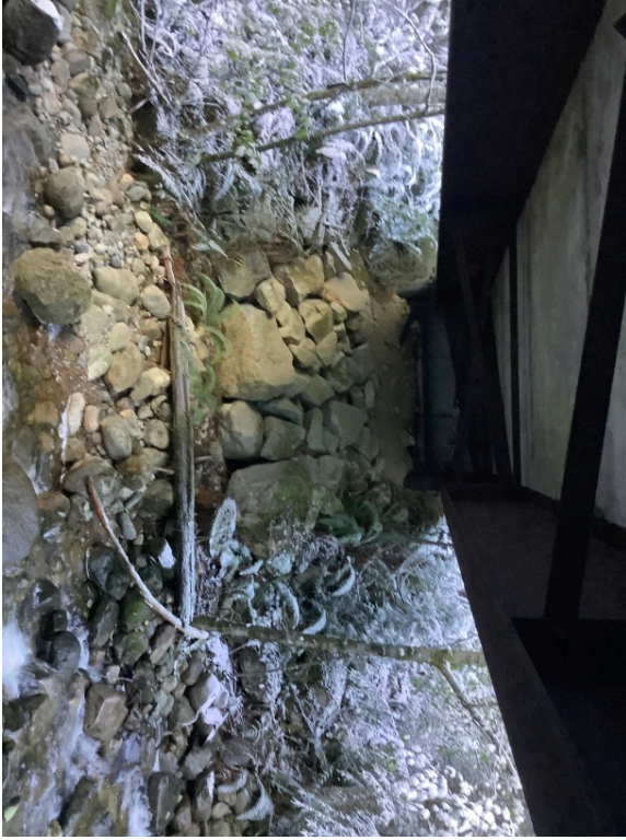
Right Bank Abutment when facing downstream
